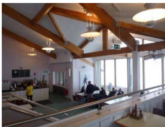
2.1b – Glulam roof beams in lieu of steelwork.
