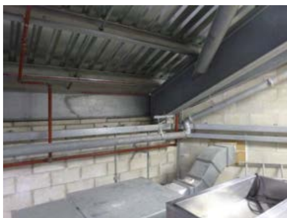
2.1a – Galv roof steelwork, non loadbearing block, bracing.
