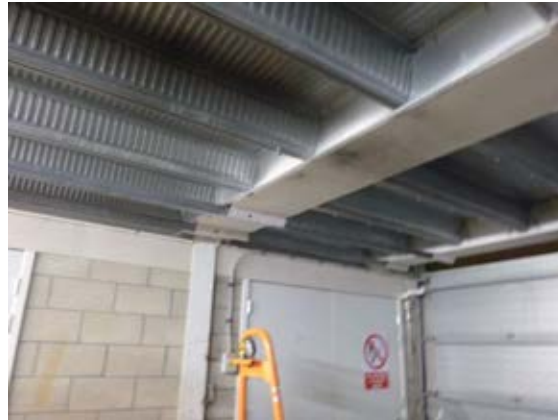
2.1d – Typical composite floor on steel frame.
